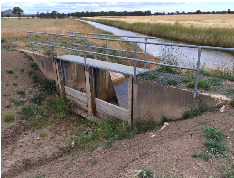
Wimmera Inlet Channel Loop Channel
