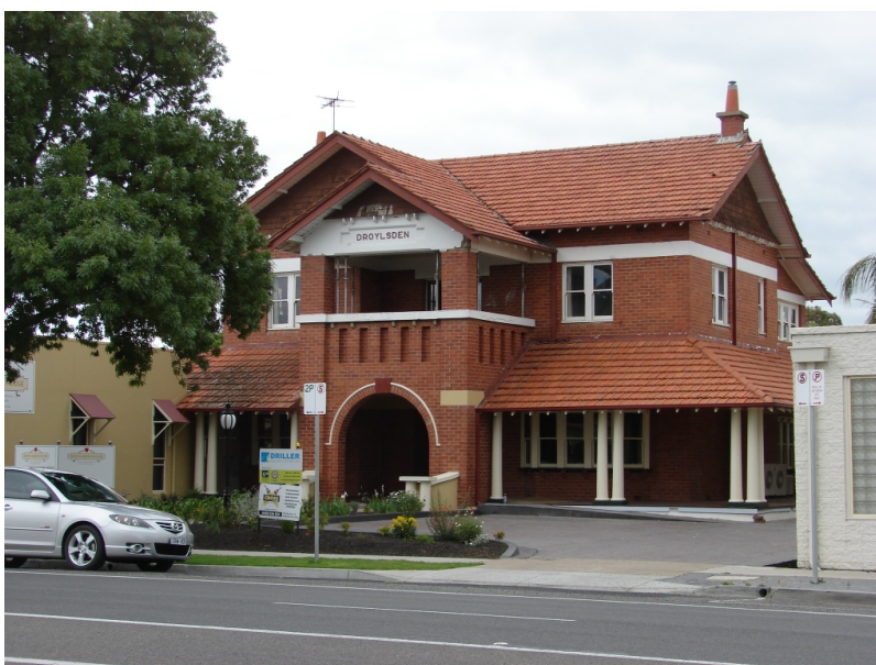
'Droylsden', 143-145 Baillie Street Horsham
