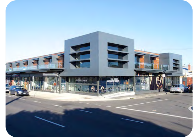
Ground floor retail or commercial can also accommodate residential uses above.
