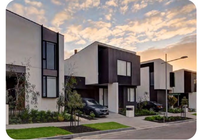
Front yard and garage positively contribute to the streetscape
