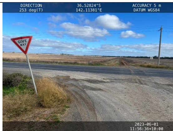
Photo 23 – Reynolds Rd: Looking west at damaged giveaway sign at Western Hwy
